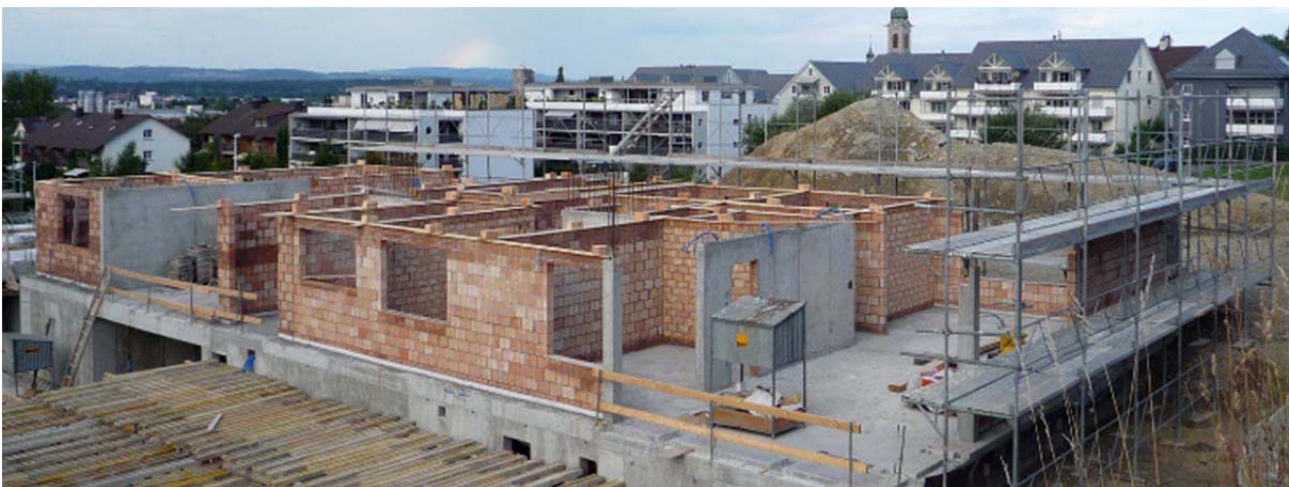
Figure 1.2: Residential building in Switzerland with RC and URM walls (Photo: T. Wenk)
