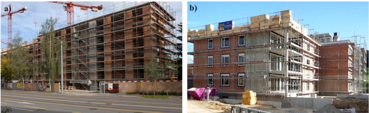
Figure 1.1: Residential buildings in Switzerland with RC and URM walls (Photos: T. Wenk)
