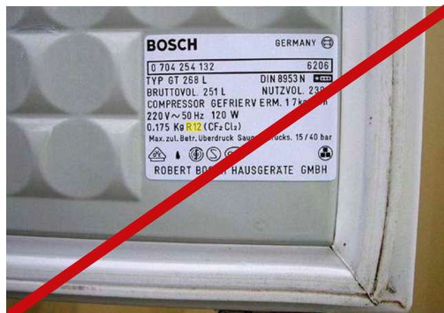
Refrigerator with forbidden refrigerant R12
