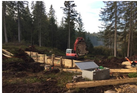
Rehabilitation work (October 2018)
