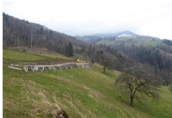
During repair work
