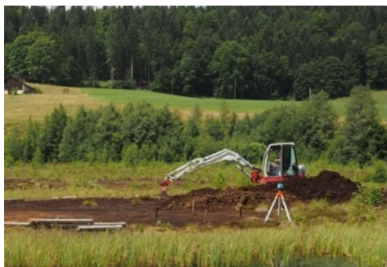
Earthworks at the Marais-Rouge in 2018
