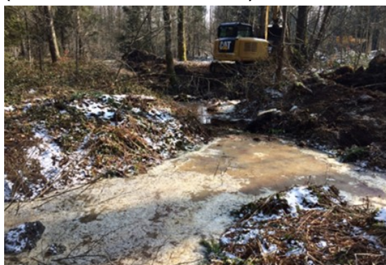
Carrying out the improvement measures
