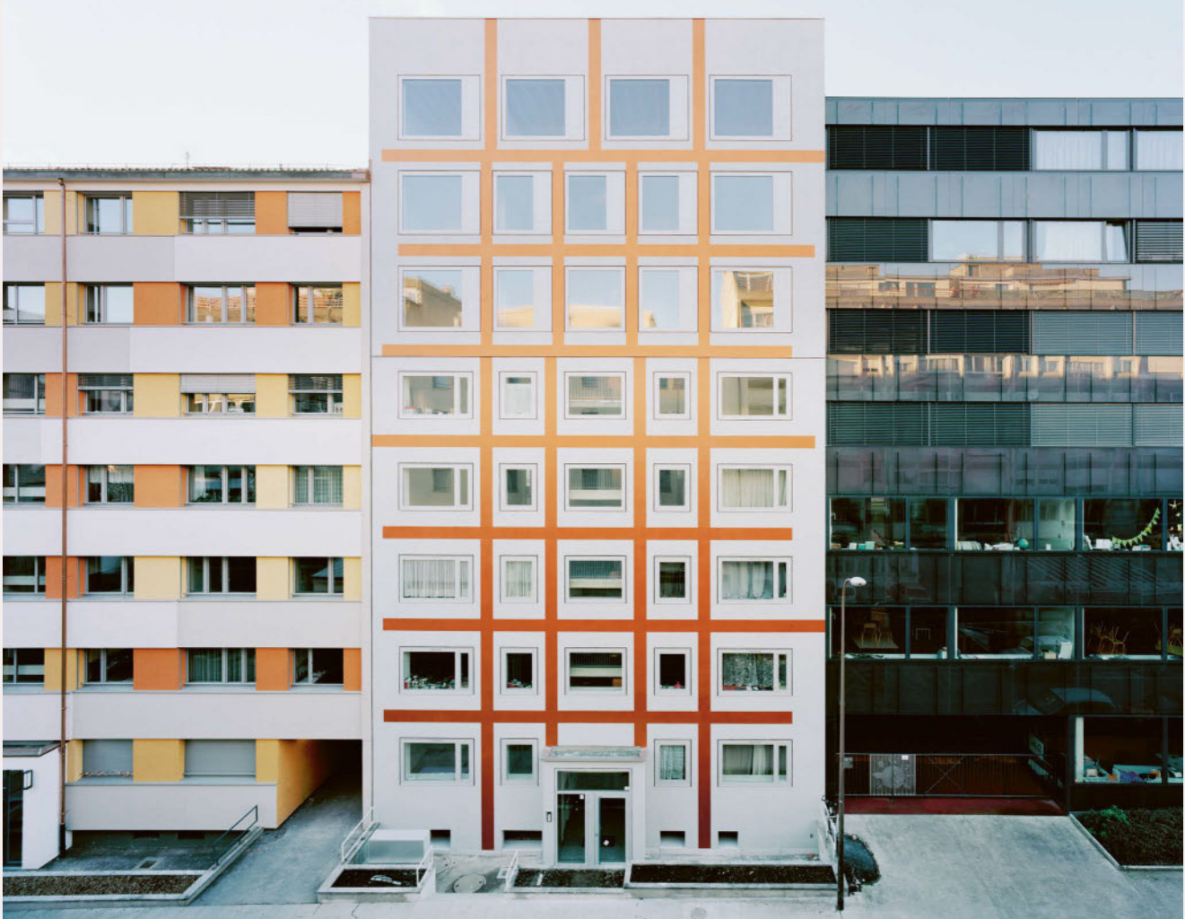
In Geneva, a project to add additional floors to the 1950s Sécheron apartment block was seen as an opportunity to improve the earthquake protection of the entire building.
