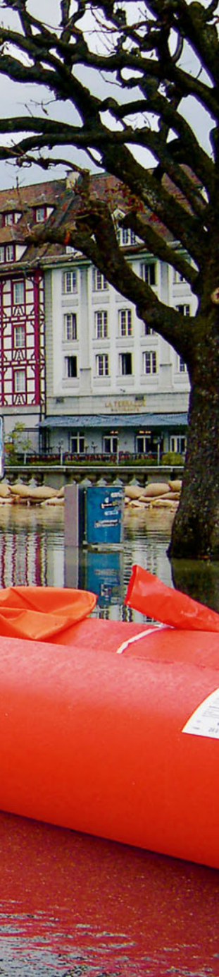
Mobile flood barriers – Beaver tubes – along the river Reuss in Lucerne.
