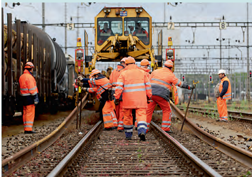
Refurbishment of railway lines: ballast and disused rails are recycled.
