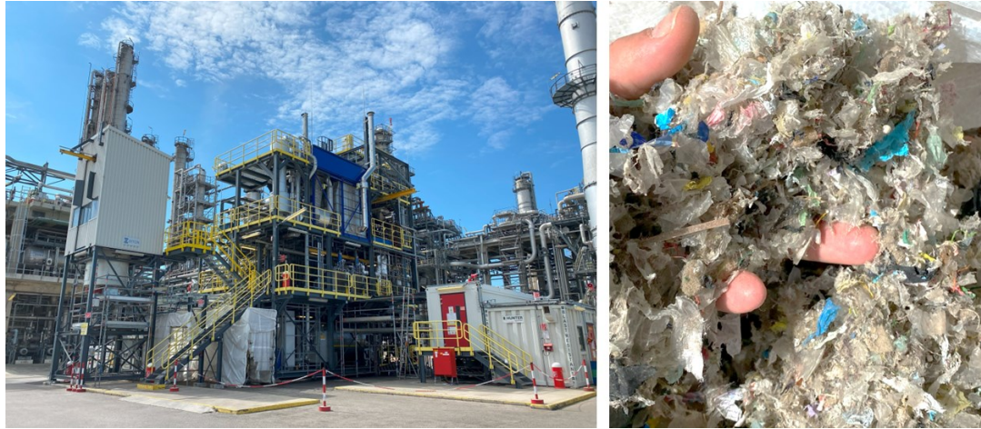
Figure 4: Pilot plant of OMV reoil-process and typical input material.
