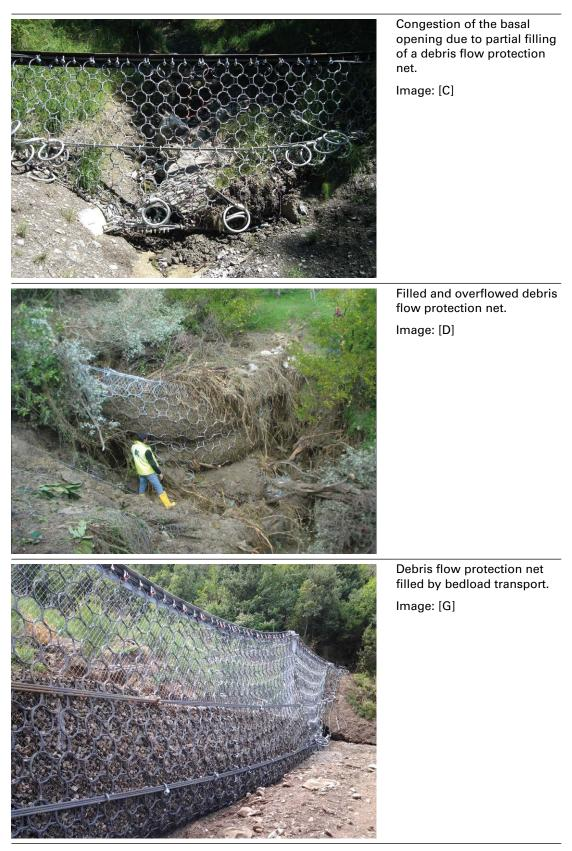
Table 8. Situation after partial or complete filling of a net barrier.
