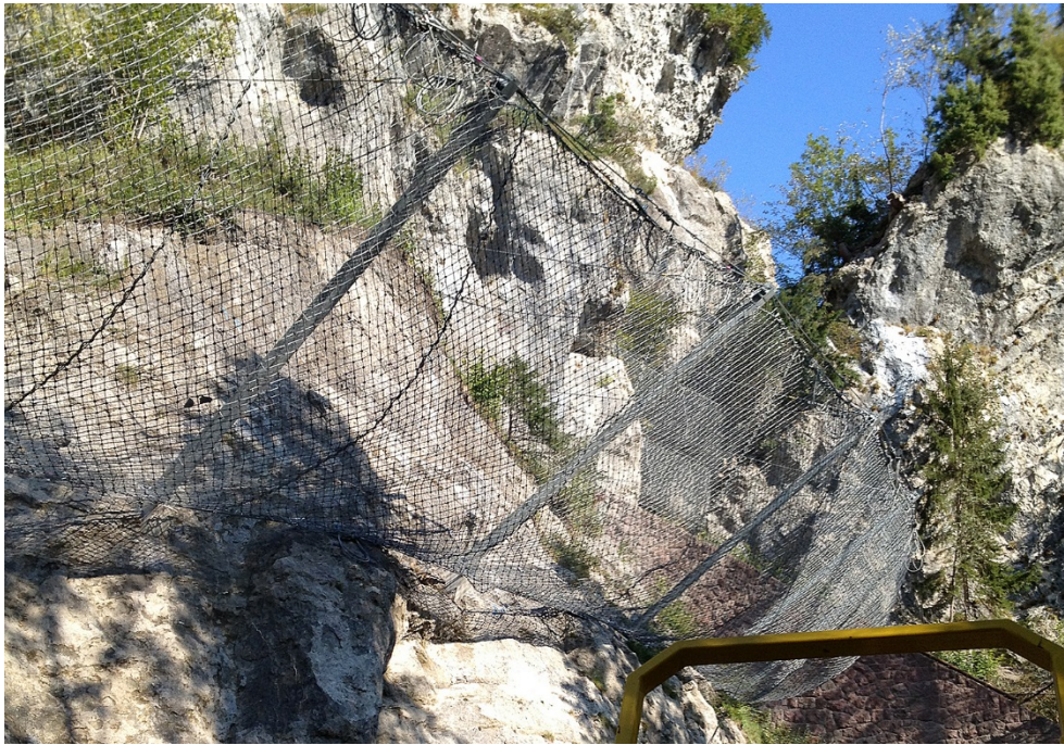
Fig. 3 > Rockfall protection net
