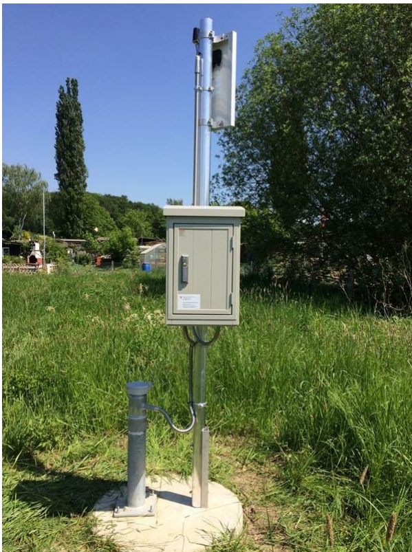
NAQUA-QUANT piezometer site for monitoring groundwater level.
