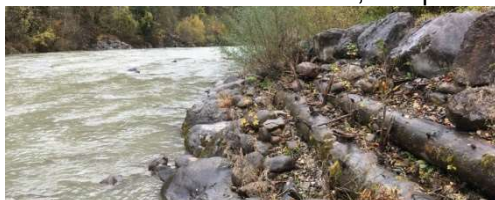
Permeable embankment, steep
