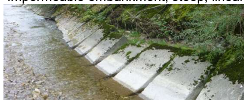
Impermeable embankment, steep, linear
