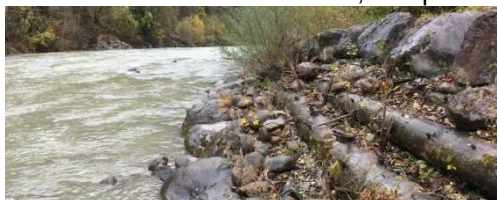
Permeable embankment, steep
