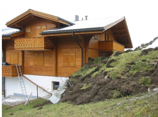
Grindelwald 2002, Photo GEOTEST AG
