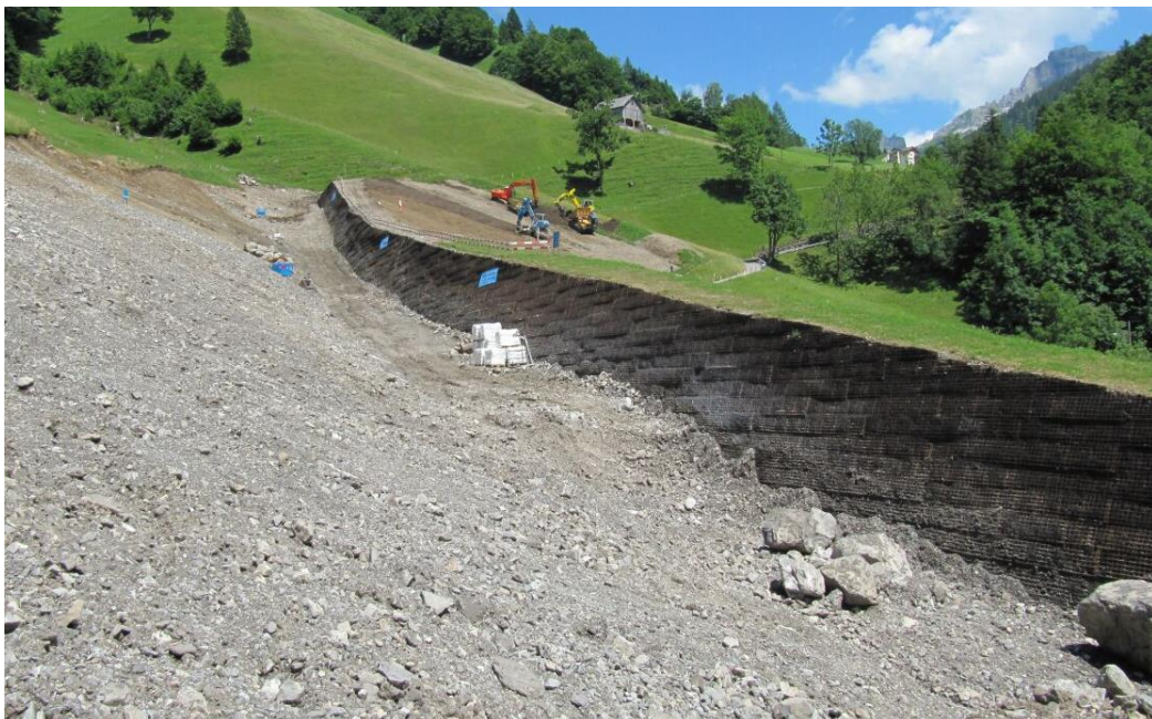
Fig. 4.4: Embankment Riemenstalden, Canton Schwyz, constructed with geogrid reinforcement, (Photo: B. Kister, 2015)
