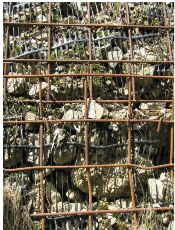
Fig. 4.9: Example of an embankment constructed with geogrid reinforcement on both slopes nearby Lecco, Italy (Photos: B. Kister).
