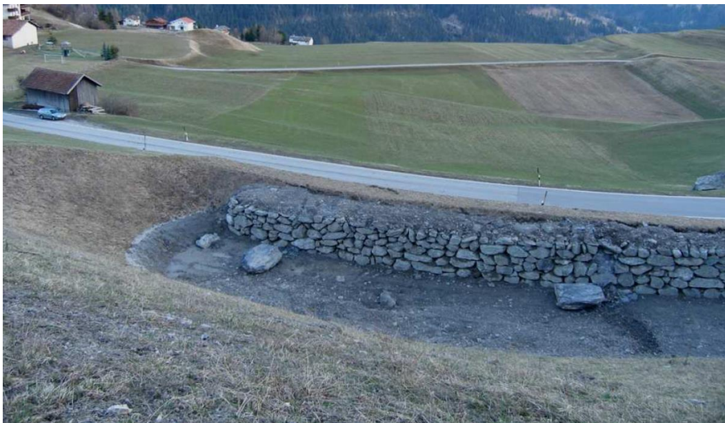
Fig. 4.3: Impacts of two blocks ( 4 \text{ m}^3 resp. 6 \text{ m}^3 ) in 2011 at embankment Gretla after redesign and implementation of rockery at the uphill slope (Photo: Tiefbauamt Graubünden). The rockery showed only minor damage.
