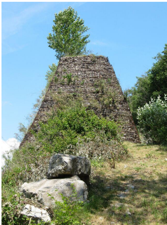
Fig. 4.9: Example of an embankment constructed with geogrid reinforcement on both slopes nearby Lecco, Italy (Photos: B. Kister).
