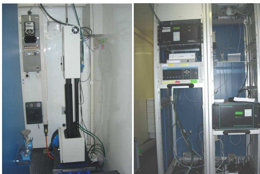
Fig. 3.1: Inside the measurement container.
