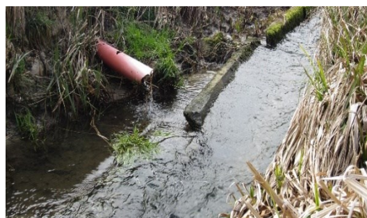
Figure 9 Photo de drainage agricole (Zaugg 2020)
