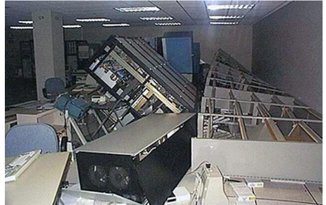
Abb. 2.21.2 > Umgekippte Computerracks
