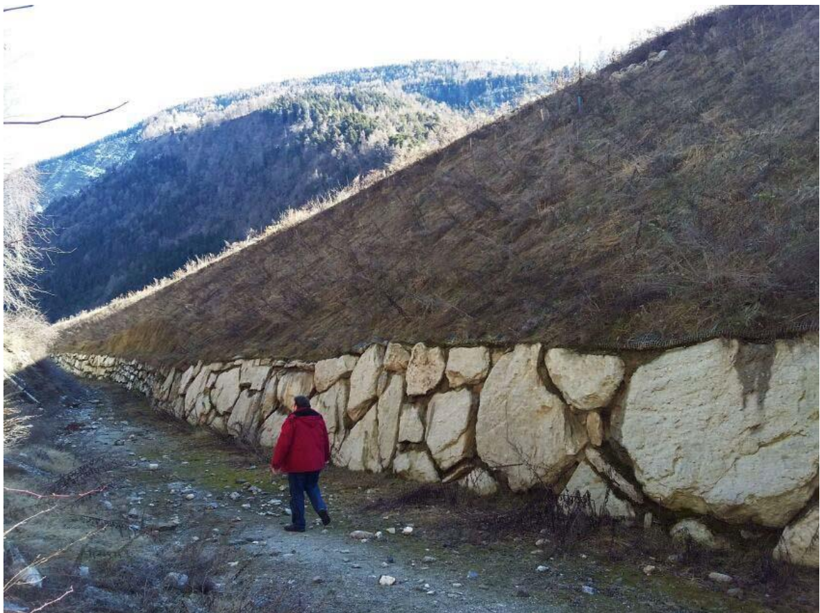
Fig. 1.4: Example of a rockfall protection embankment in Canton Valais with rockery placed in the lower part and soil at the upper part of the uphill slope. The surface roughness of the rockery may be described as smooth and is comparable with the surface roughness in Fig. 1.3a) and c) (Photo: S. Lambert).
