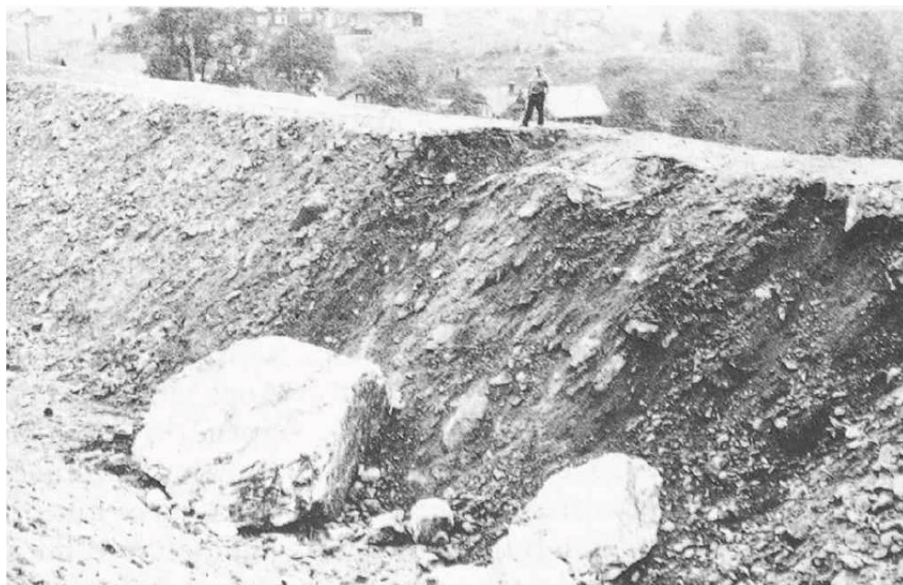
Fig. 4.2: Impact at the embankment Halteli-Talmatt, Canton Uri. The embankment was neither punched through nor surmounted, but the impacting block reached the crest (Schneider, 1984)
