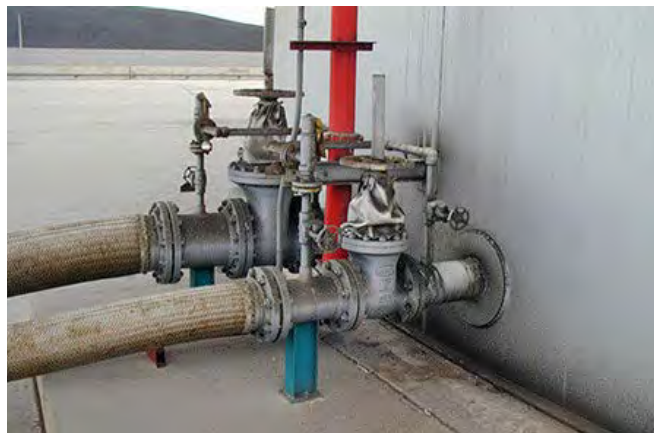
Fig. 2.17.6 > Raccords flexibles
