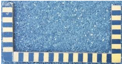
Wassen, Gotthardstrasse SDA 4 2016
