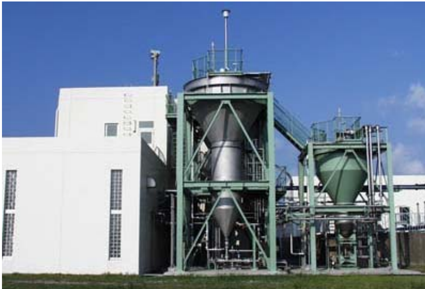
Abb. 28 > PHOSNIX Anlage im Lake Shinji Eastern Clarification Center der Shimane Prefecture (SECC)
