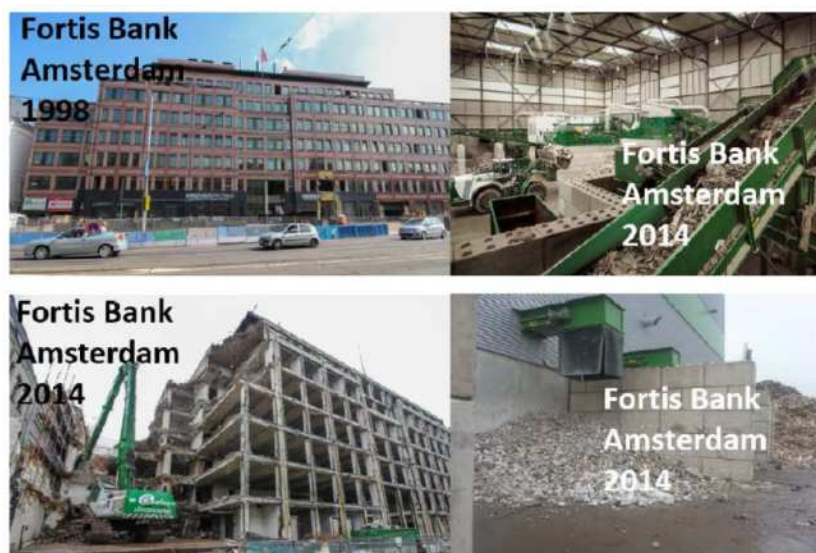
Figura 5 Stato dell'edificio Fortis Bank Amsterdam. Fonte: Deliverable D8. Reversible Building Design. Reuse Potential Tool. Elma Durmisevic et al. BAMB. February 2019
